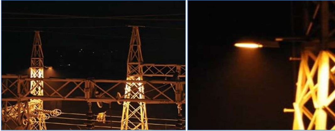
Plate 7: Down-facing lights at the port reduce sky glow
