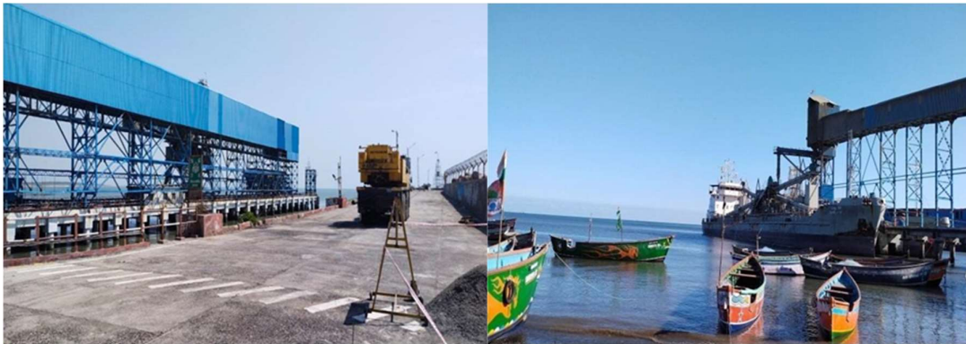
Plate 1: View of Project Site
