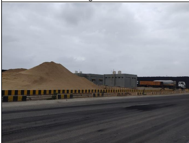
Sulphur Storage Plot
