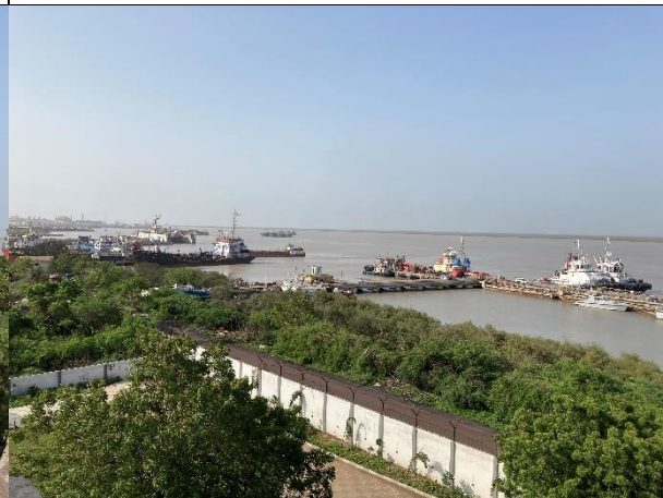
Salvage and Navigation Aid Jetty
