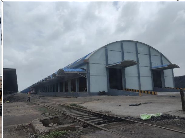
Dome Shape Storage Shed
