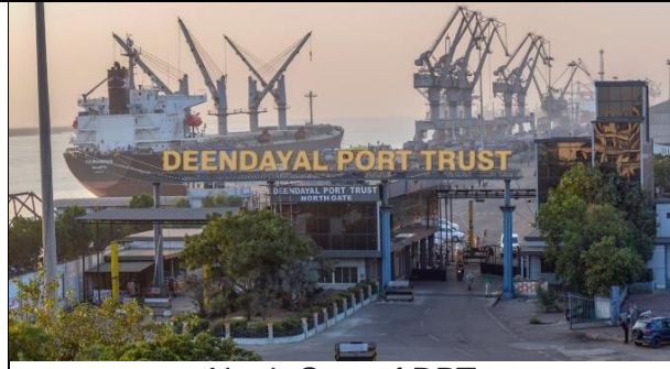
North Gate of DPT
