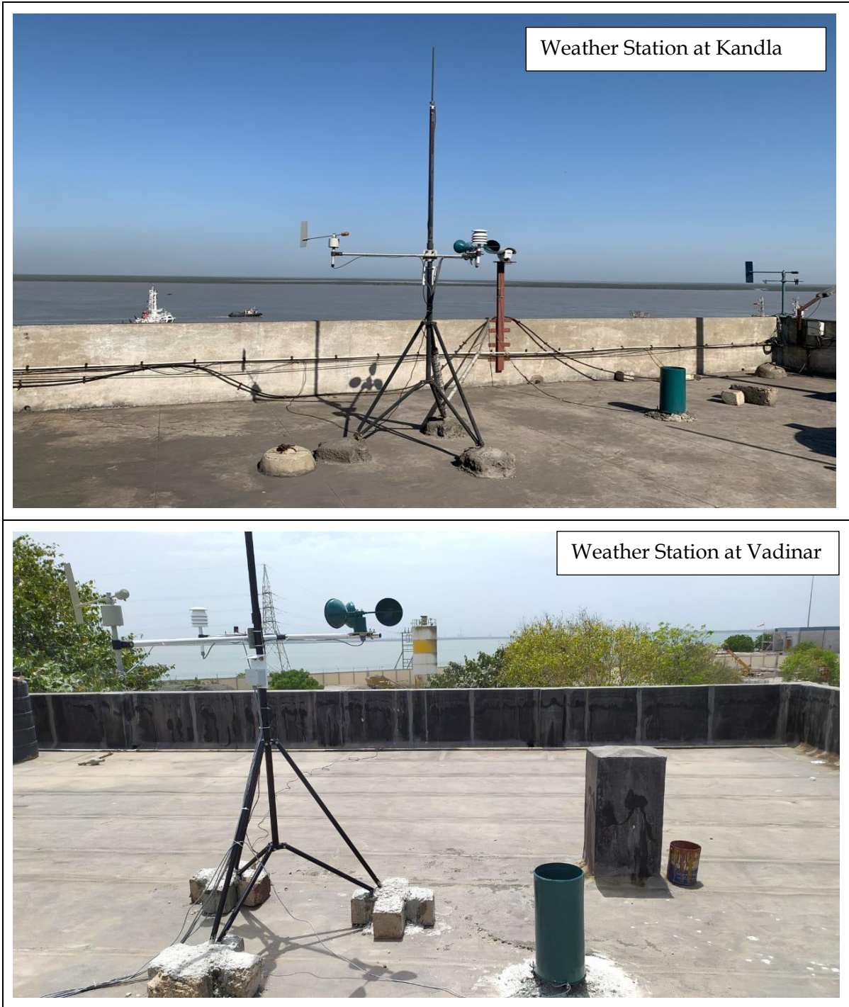
Figure 2: Photographs of Automatic Weather Monitoring Station at Kandla and Vadinar
