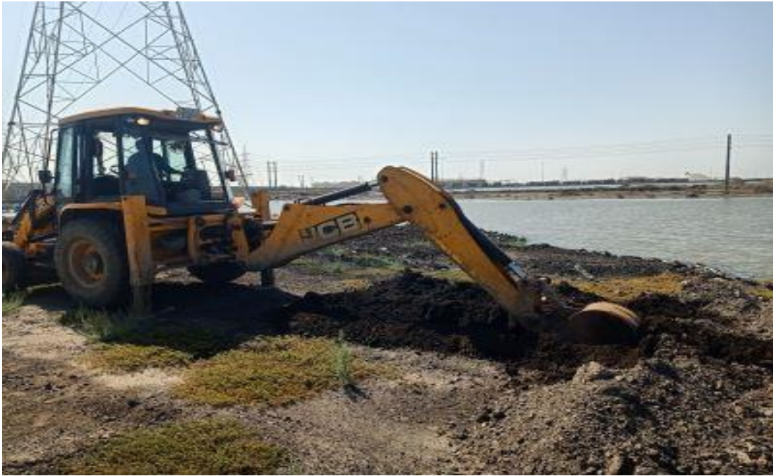
Digging Out the Trench Through JCB
