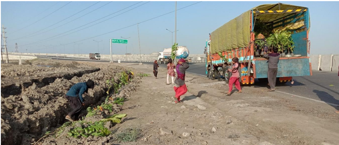
Fig. 5 Transportation of Plants to Site
