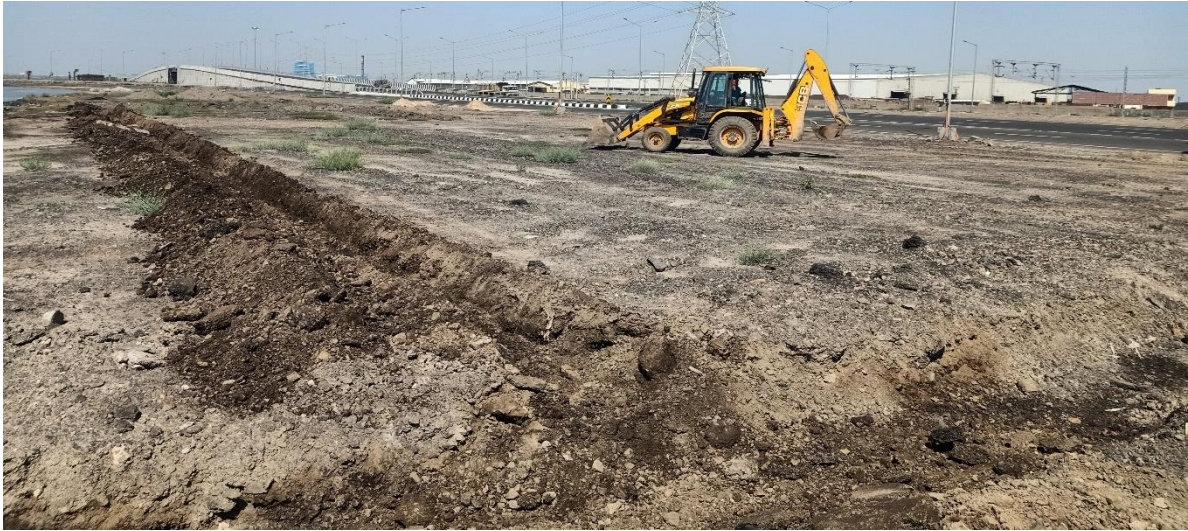
Fig. 4 Digging Out Trench for Plantation
