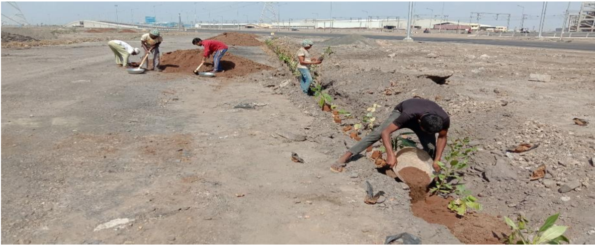
Fig. 7 Soil Filling in Plantation Pits
