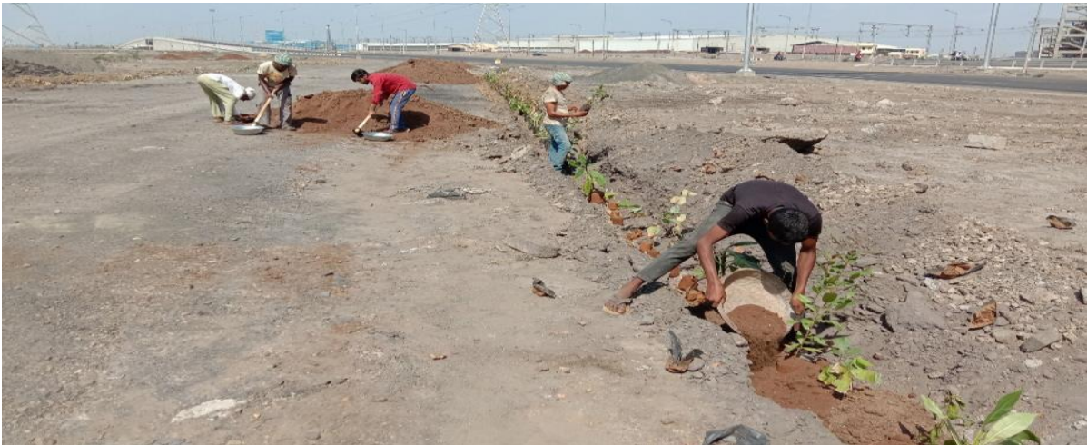
Fig. 7 Soil Filling in Plantation Pits
