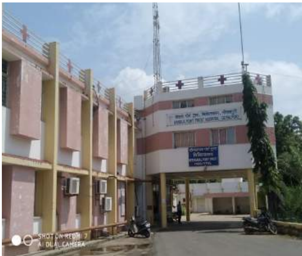
Figure 13: Gopalpuri hospital at Gandhidham
