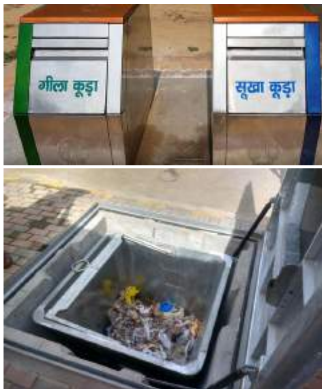
Figure 9a: Smart underground roadside bins
