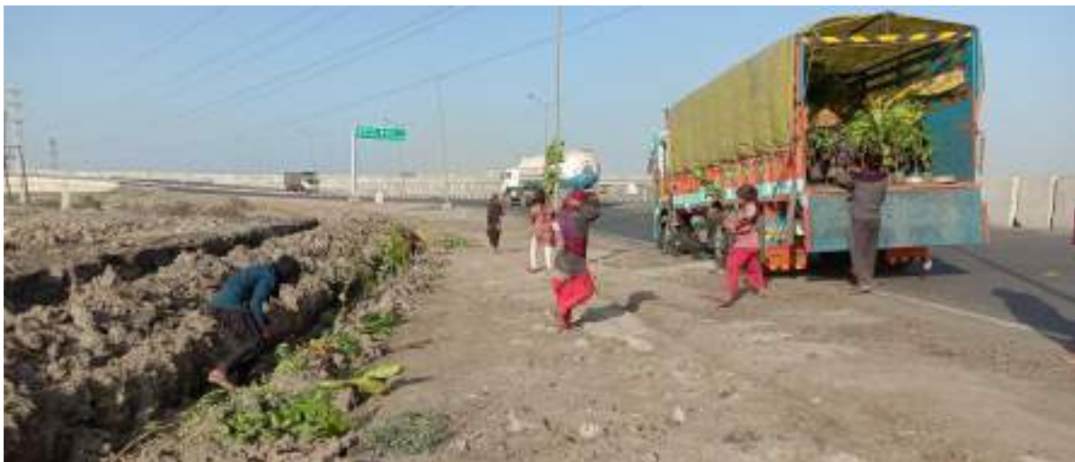
Fig. 5 Transportation of Plants to Site
