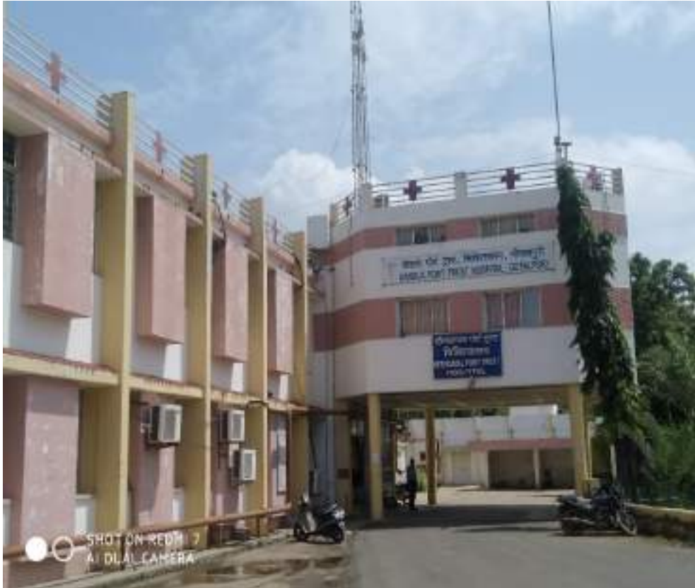
Figure 13: Gopalpuri hospital at Gandhidham
