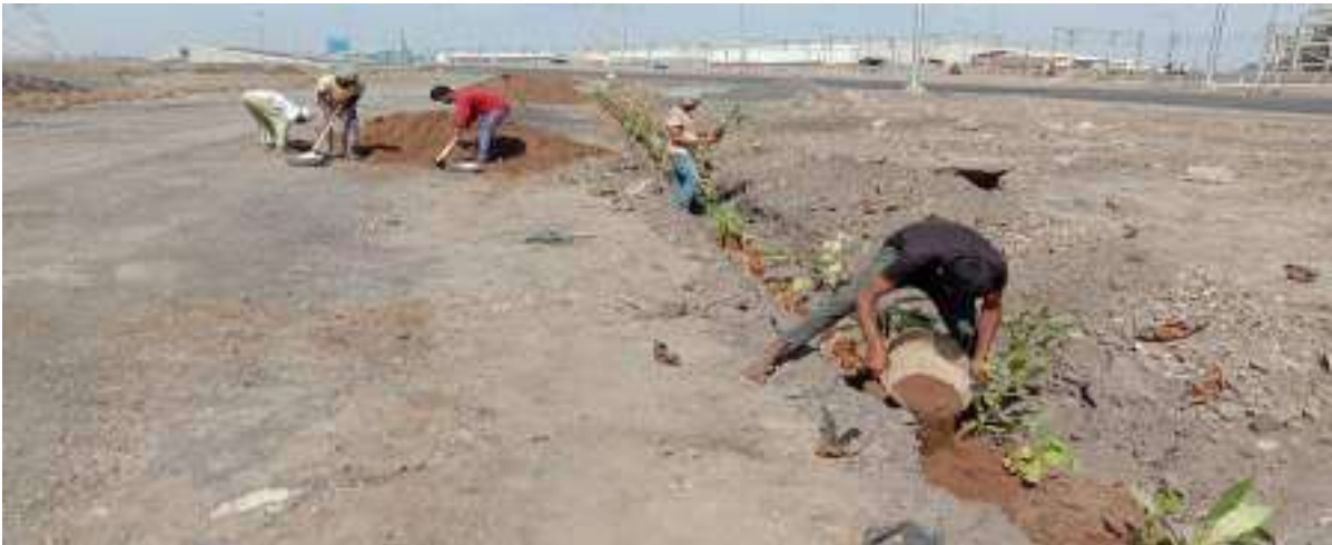
Fig. 7 Soil Filling in Plantation Pits
