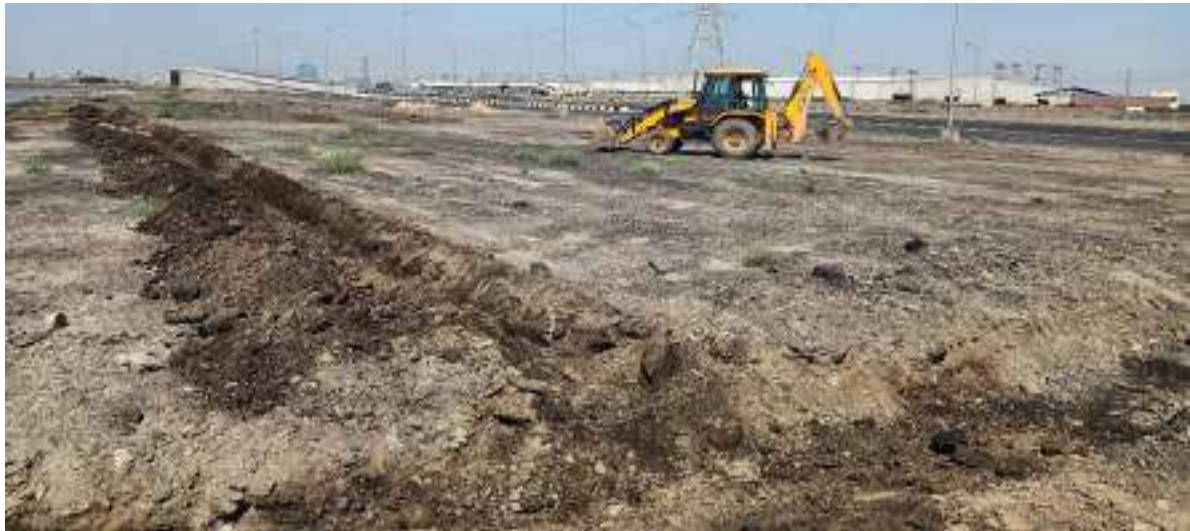
Fig. 4 Digging Out Trench for Plantation
