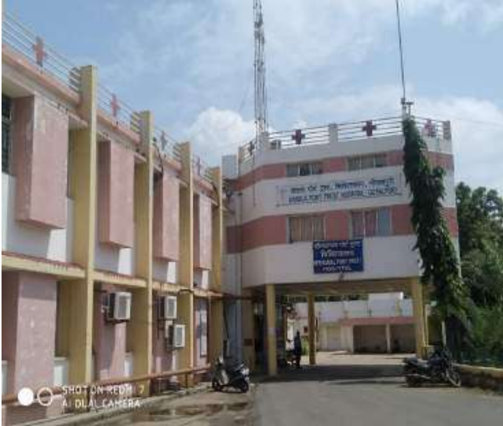
Figure 13: Gopalpuri hospital at Gandhidham
