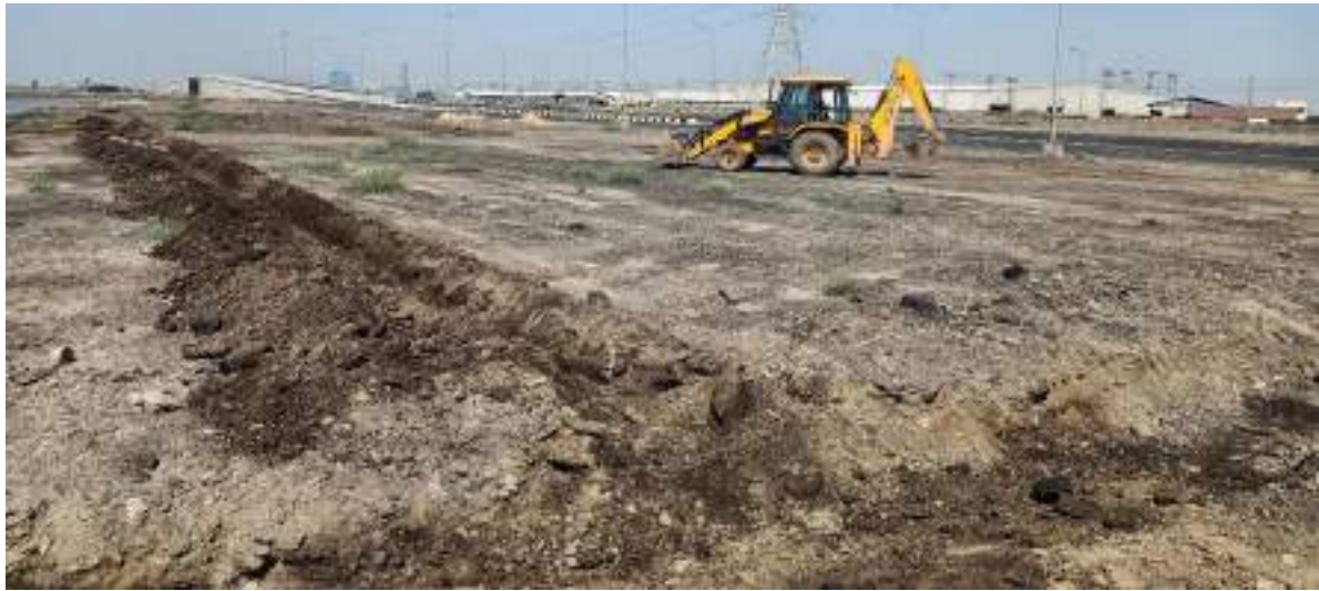
Fig. 4 Digging Out Trench for Plantation
