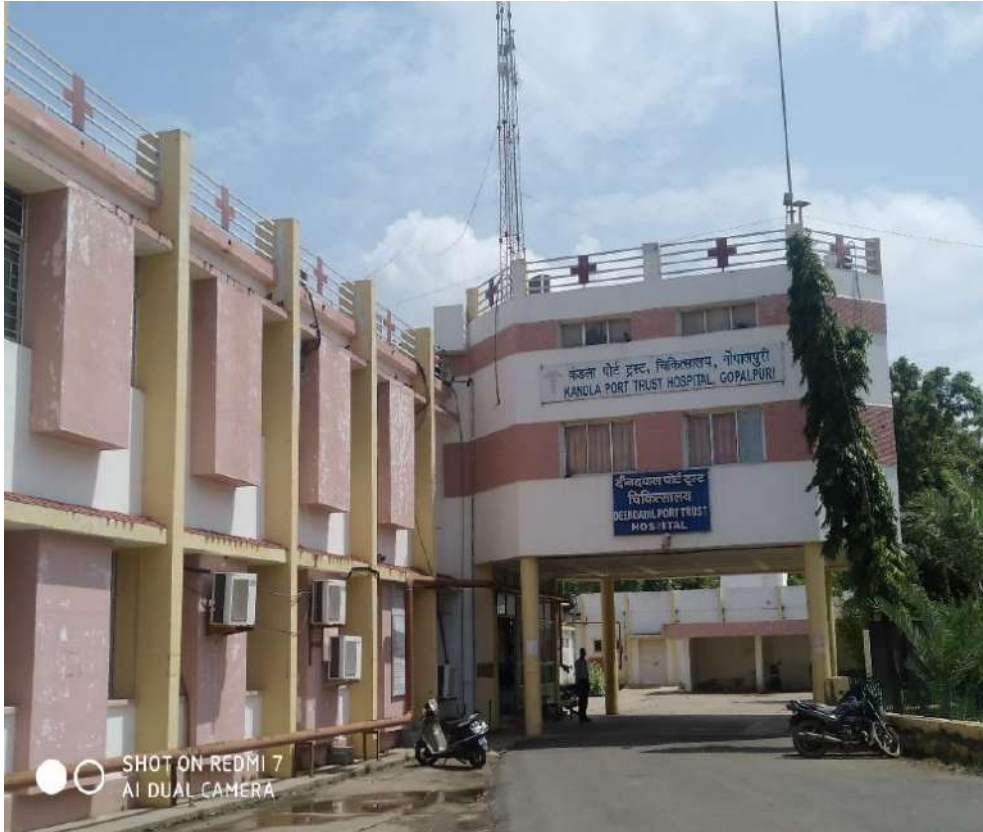
Figure 13: Gopalpuri hospital at Gandhidham
