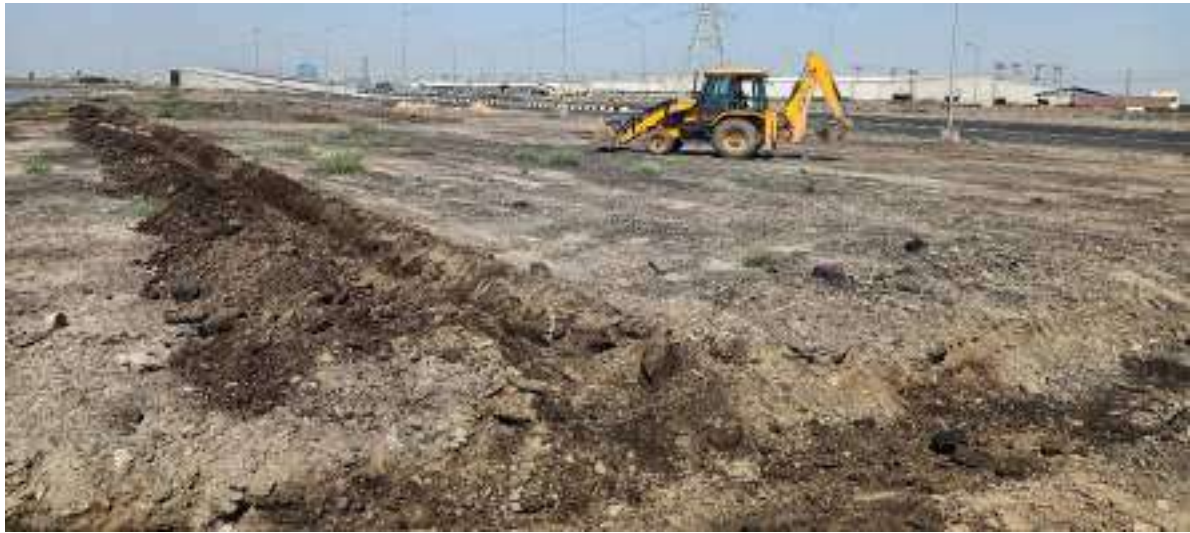
Fig. 4 Digging Out Trench for Plantation
