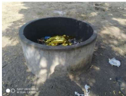
Figure 3: Concrete bins at Gopalpuri colony campus, Gandhidham
