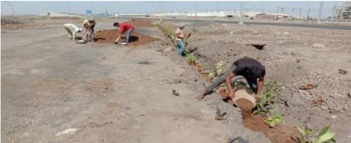
Fig. 7 Soil Filling in Plantation Pits
