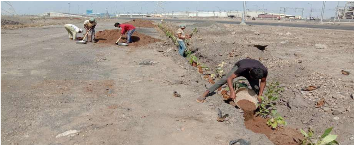
Fig. 7 Soil Filling in Plantation Pits
