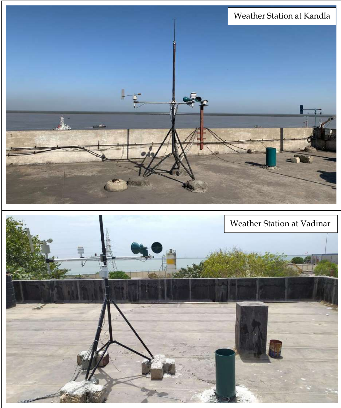
Figure 2: Photographs of Automatic Weather Monitoring Station at Kandla and Vadinar
