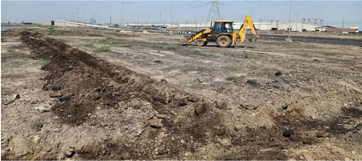
Fig. 4 Digging Out Trench for Plantation
