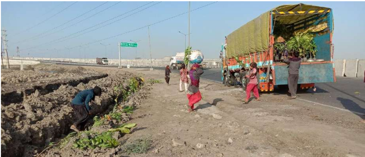
Fig. 5 Transportation of Plants to Site
