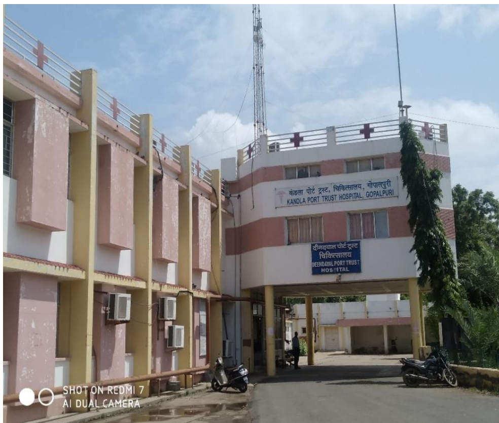
Figure 13: Gopalpuri hospital at Gandhidham
