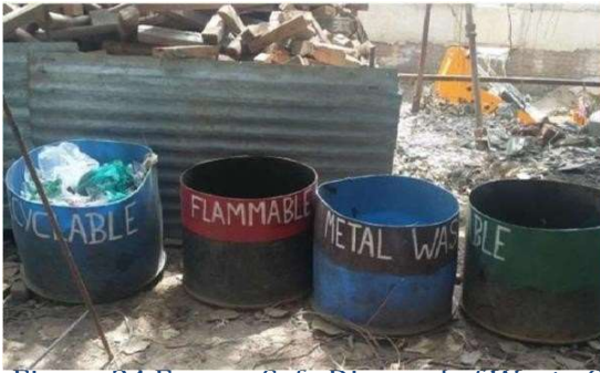
Figure 24 Ensure Safe Disposal of Waste Generated During Construction various construction waste
