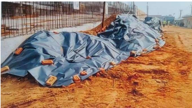
Figure 19 Covering of fine aggregate and excavated earth on site
