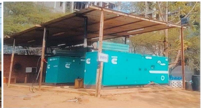
Figure 30 Ensure diesel generator sets are in compliance with CPCB norms and have an exhaust with stack height of at least 2 m from the top of the generator with a cap.
