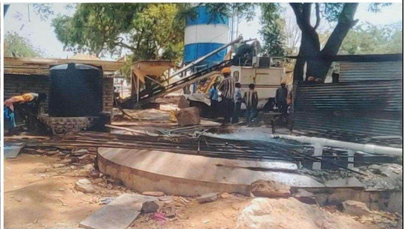
Figure 14 THIS IS NOT ALLOWED Construction Waste Improperly St
