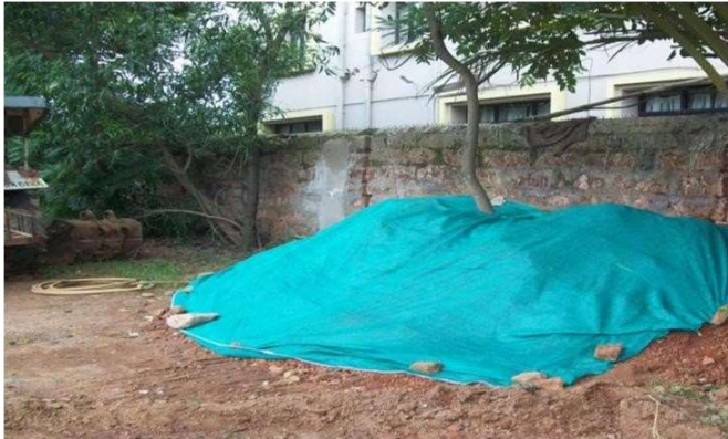
Figure 5 30 cms of Topsoil to Be Stacked in the Layer of 40 cms And Covered with Green Net to Prevent Soil Erosion
