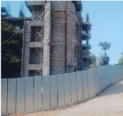
Figure 16 3m High Continuous Impervious Barricading Along the Site Virtual
