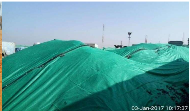
Figure 20 Covering of fine aggregate and excavated earth on site
