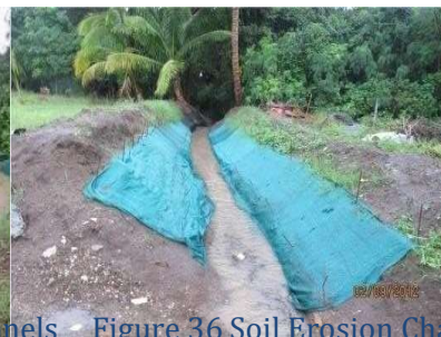
Figure 36 Soil Erosion Channels
