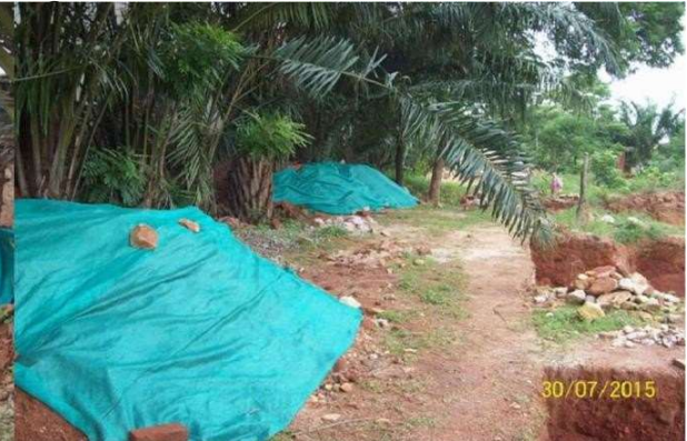
Figure 6 30 cms of Topsoil to Be Stacked in the Layer of 40 cms And Covered with Green Net to Prevent Soil Erosion
