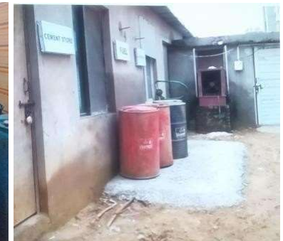
Figure 23 - Correct practices - spill prevention plan
