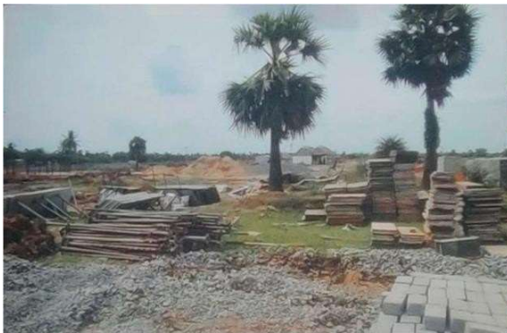
Figure 12 Bad Example of Stacking Building Material on Site
