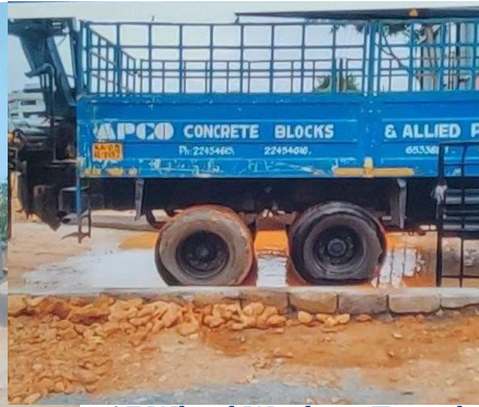
Figure 17 Wheel Washing Trough at Entrance
