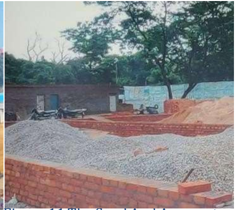
Figure 11 The Sand And Aggregates Are To Be Stored In A Way So That They Do Not Spread Over The Surroundings. Keeping Watering the Fine and Course Aggregates against Any Erosion
