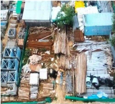
Figure 9 Good Examples of Stacking Building Material on Site
